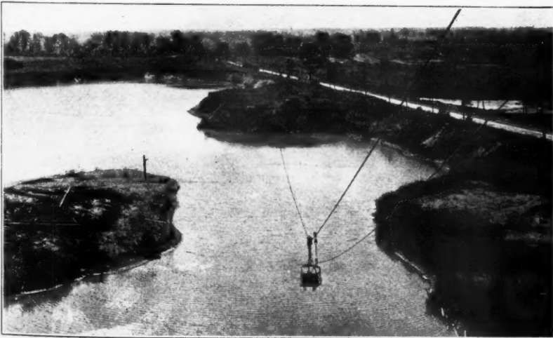
The Pit Operated By the Single Unit Cableway; Plant at Indianapolis
